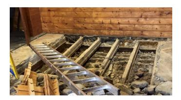
We hired a contractor to change the layout of the gym, which took 8 weeks. In the first week of the construction our contractor dug up the floor to replace the concrete with industrial standard, which is able to resist the heavy weights dropped during our sessions. The next step was to dig up the floor on the outside of the door to be able to make the whole gym surrounded evenly by four walls. In the second week the concrete was filled in the floor and excess wood from the inside thrown away.
